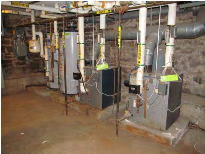
Original boilers for production of hydronic heat with newer freestanding domestic hot water tanks in background
