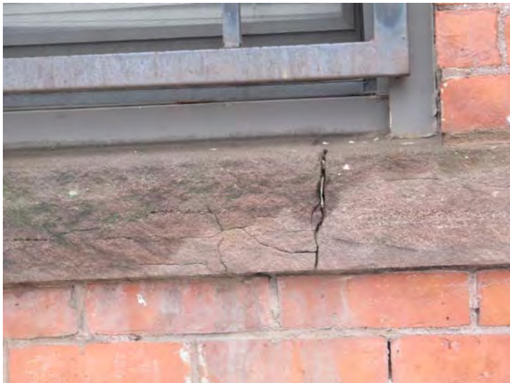
Cracked brownstone window sill
