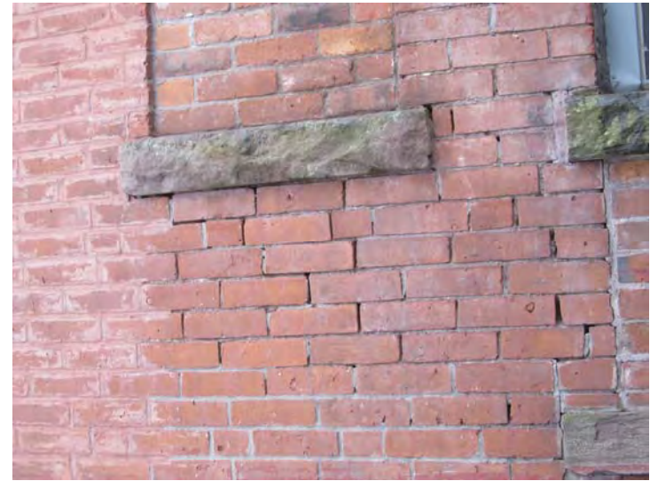
Brickwork in need of repointing also evident at various locations
