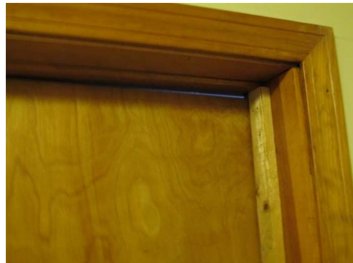
Entry doors to units from common halls exhibit past repair efforts and gaps around the frame
