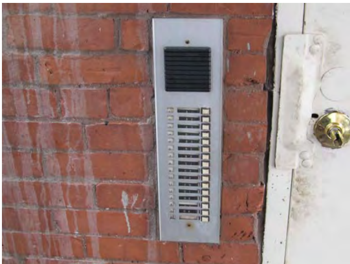
Door buzzer/intercom panels are at or near the end of their expected useful service lives
