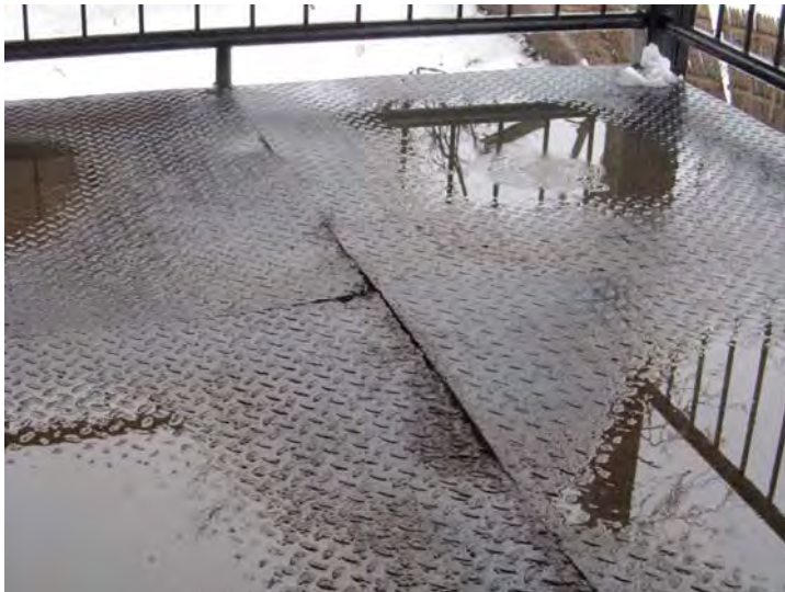
Worn/uneven areas of steel decking noted at various locations on landings of rear stair assembly
