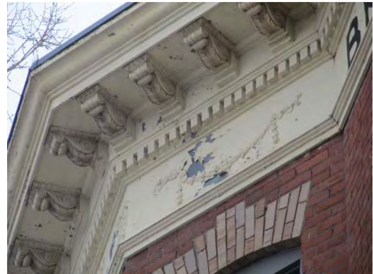
Metal cornicing at front elevation in need of surface preparation and painting
