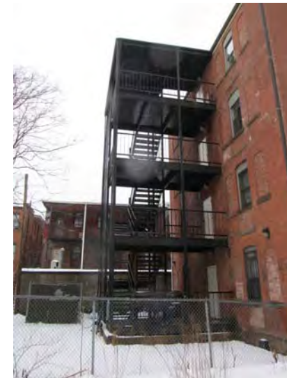
Building architecture at rear elevation features multi-story steel stair/fire escape assembly
