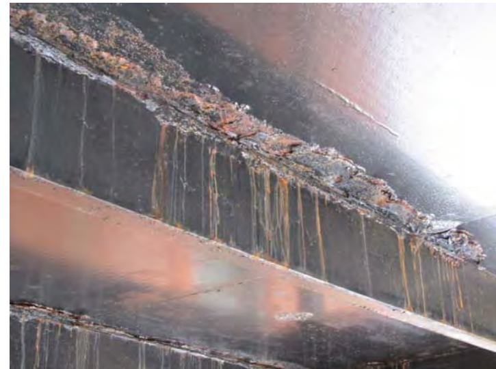
Rust damage also visible on underside of steel decking
