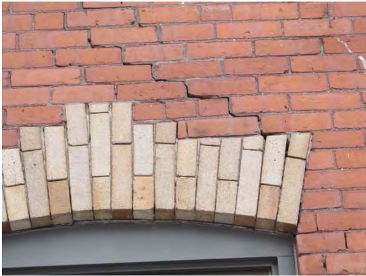
Cracks noted in brickwork at various locations
